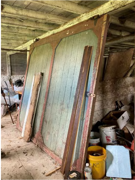
Figure 3 – One of the west barn doors.
