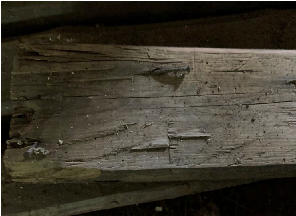
Figure 2 – Timber barn member showing hand-hewn adze marks.
