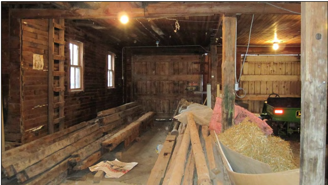
Interior of west section. (Paul Bergson photographs) Top: Second floor. Bottom: First floor.
