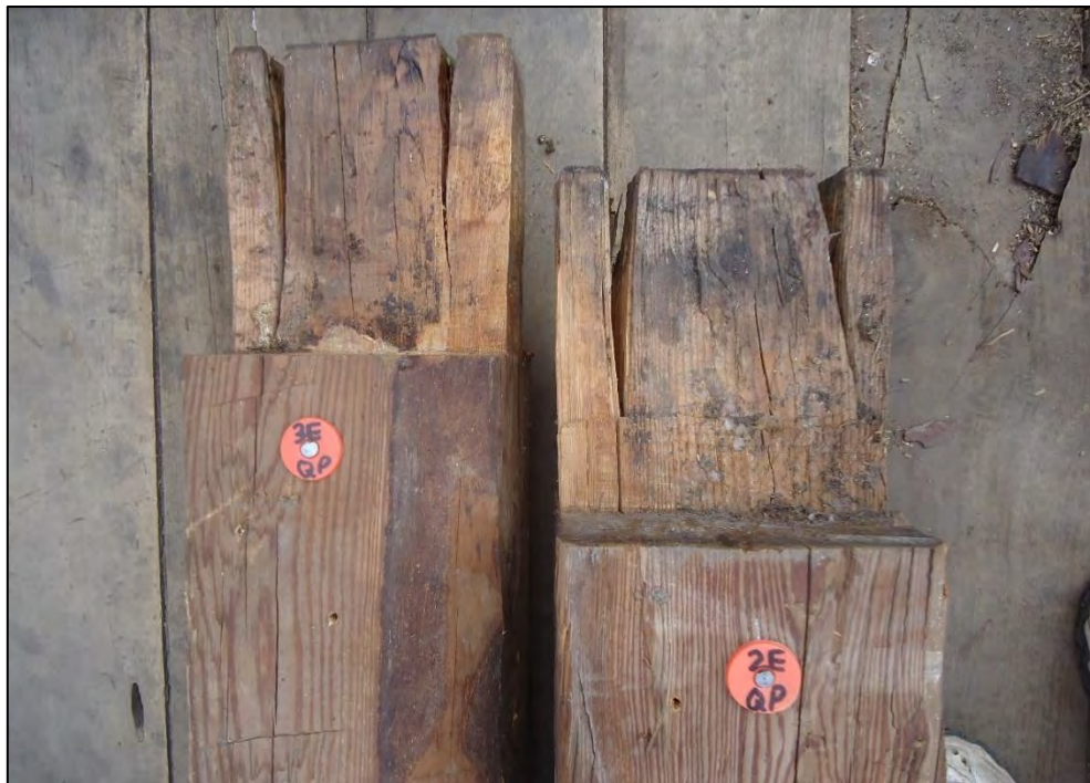
Labeled structural members. (Curt Richter photograph)
