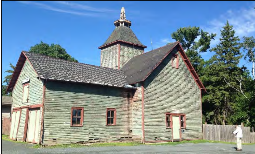
Photographs before barn was disassembled.
