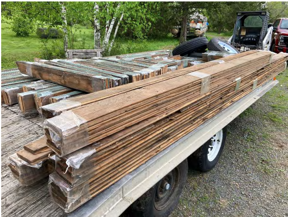
Figure 10 - Clapboard siding and interior sheathing boards on trailer.
