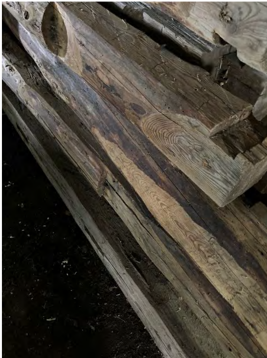
Figure 5 – Timber members showing hand-hewn notches.
