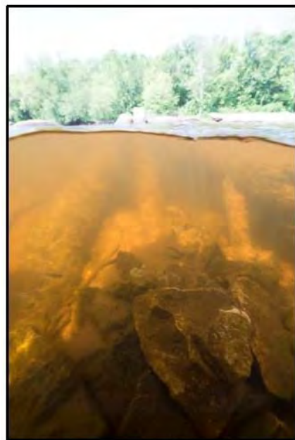
FIGURES 49-54. Images showing details of the large dam at Boom Island.
