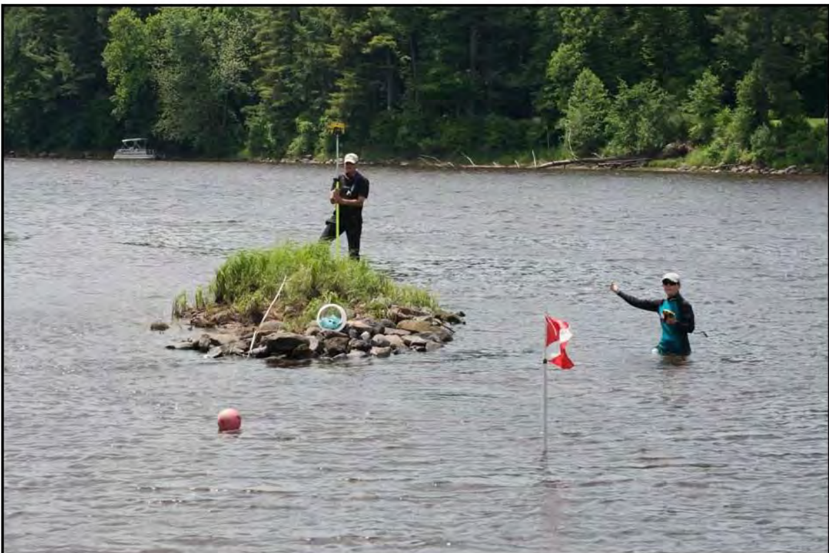
FIGURES 89 and 90. Images from Log House Landing brush and rock dam.
